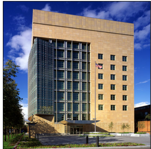
Moscow, Russia, NEC. Architect: Hellmuth Obata + Kassebaum Photo: HOK
