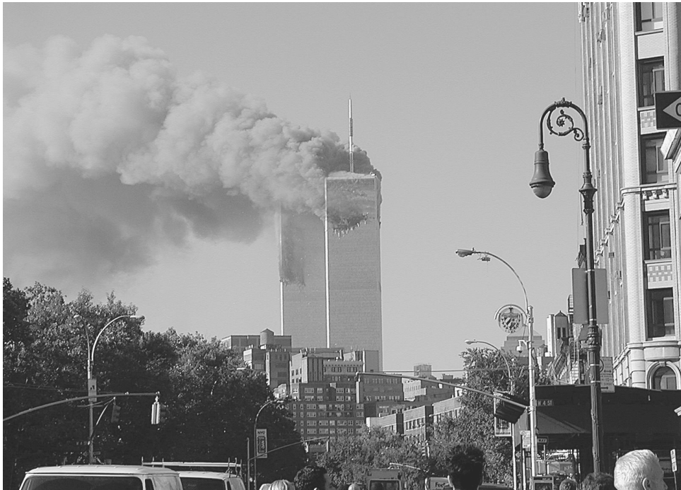
FIGURE 1.1 World Trade Center towers on September 11, 2001, at 9:05 a.m., looking south from 6th Avenue and Washington Place, New York, N.Y. (Architect: Minoru Yamasaki with Emory Roth and Sons; photographer: Bruce D. Eisenberg, AIA.)
